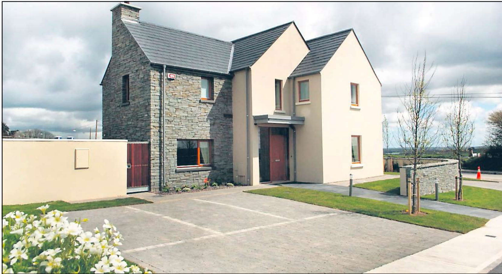
Barleyfield, Whitechurch, raises the bar for new developments all over the region.
